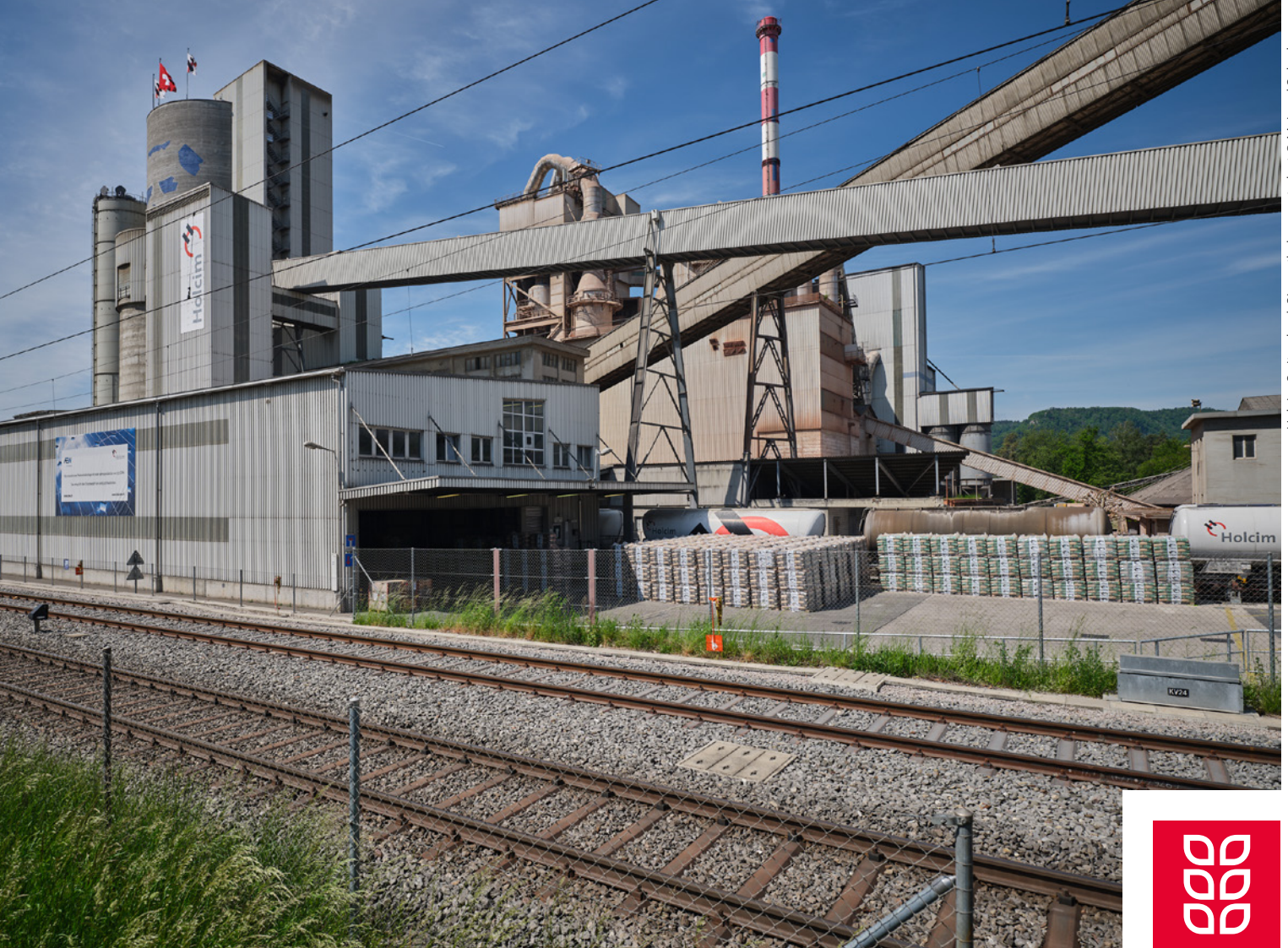
Holcim Switzerland, Siggenthal cement plant © Meinrad Schade
